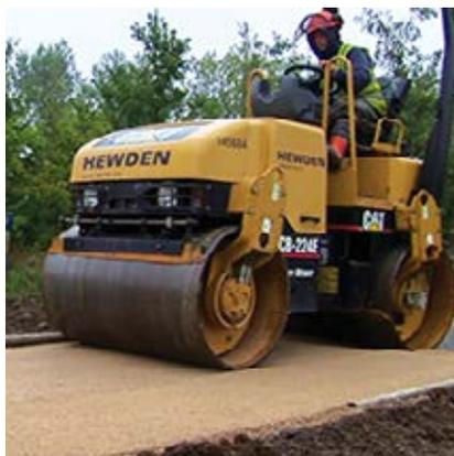
By using a heavier roller, this helps achieve maximum compaction with fewer passes, however on smaller areas a pedestrian roller may be used although it is vital that the surface is rolled sufficiently to achieve fullest compaction prior to water rolling. This may take a few more passes over the area. The sub-base should be laid with cross falls or cambers prior to the application of the Breedon Golden Amber surface course.
