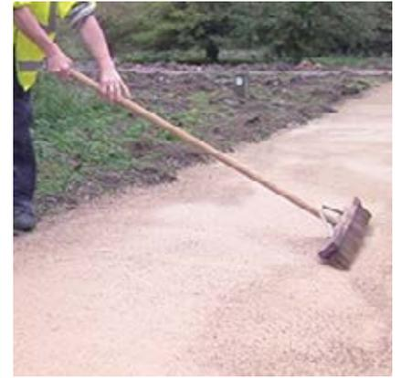
that occasional coarse areas will be evident where segregation of the Breedon Gravel may have occurred. At this point, fines can be sieved from the main heap of material and scattered onto these coarse areas before being re-rolled.
