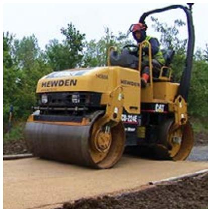
a pedestrian roller may be used although it is vital that the surface is rolled sufficiently to achieve fullest compaction prior to water rolling. This may take a few more passes over the area. The sub-base should be laid with cross falls or cambers prior to the application of the Wayfarer surface course.
